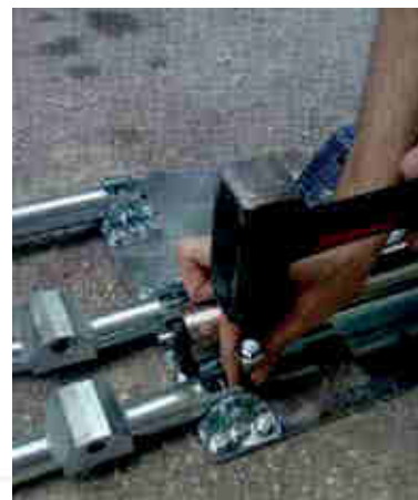
Figure 10 - Anchor placement
