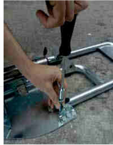
Figure 11 - Fixing the barrier
