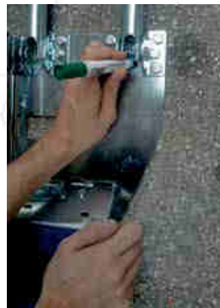
Figure 8 - Marking drilling spots
